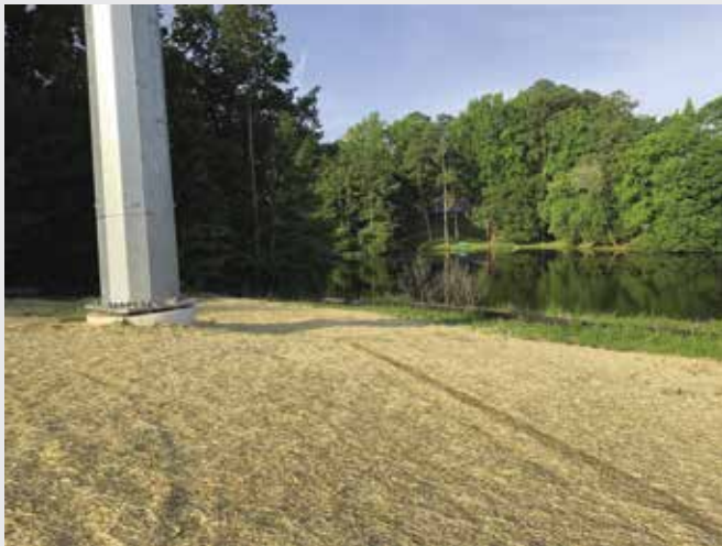
▲ Work pad stabilized with seed and straw after construction was completed. Photo courtesy of ECI.
