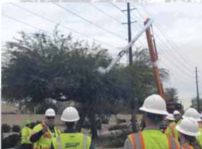
Asplundh GF Eric Juedes explaining safety precautions and proper clearances, while Dominic Garcia (in bucket) prunes a mesquite (Prosopis spp.) underneath sub-transmission and distribution lines. (Photo submitted by Pat Paternostro)
