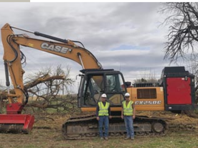
Operations Manager Blaine Flory (left) and Project Manager Mark Flory (right).
