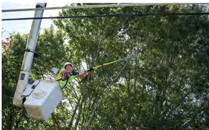
The MAD saw can also be used by workers in mechanical lift buckets, making them a versatile and easy-to-use solution for vegetation maintenance. Photo courtesy of Husqvarna.
