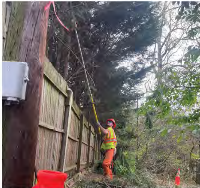
An Asplundh worker uses a MAD Saw on foot to cut back limbs. Photo courtesy of Asplundh.
