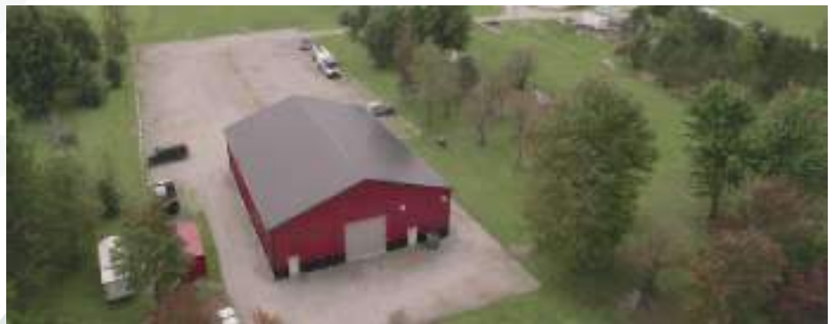
IBEW Local 17 training property in Wales, Michigan
