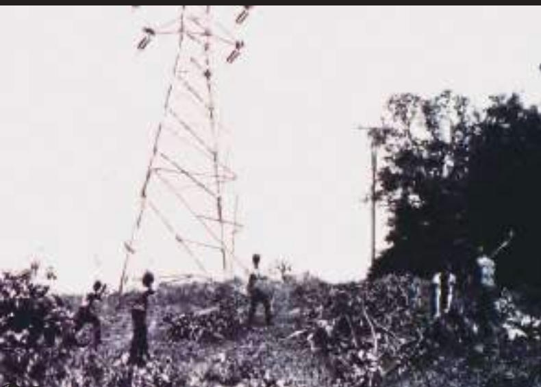
Early ROW maintenance was done largely by hand. Note the circular saw mounted on a tractor in the image on the right. Photos courtesy of Asplundh Tree Expert, LLC.
